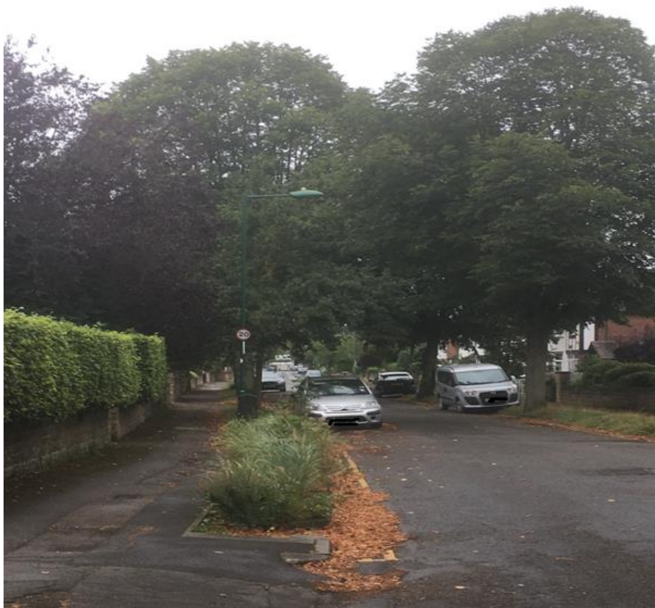
Photo of Rain Garden Ribblesdale Road, Nottingham
